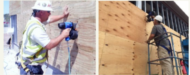
Lath to Densglass to Steel
