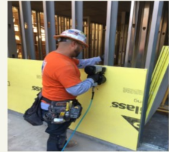
Lath & Exterior gypsum to steel framing
