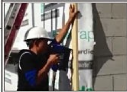
5/4" Hardie Trim to Concrete Block
