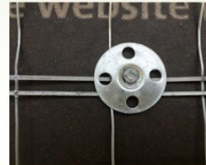
Lath & Exterior gypsum to steel framing
