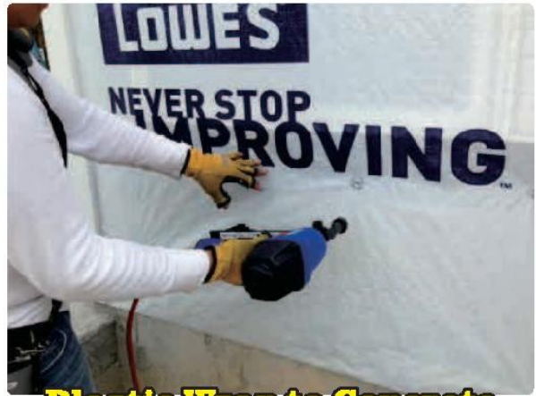
Plastic Wrap to Concrete
