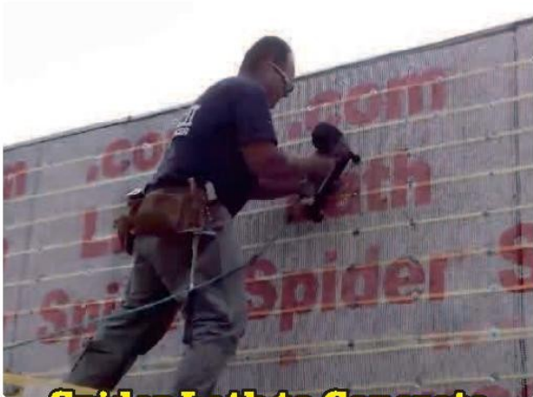
Spider Lath to Concrete
