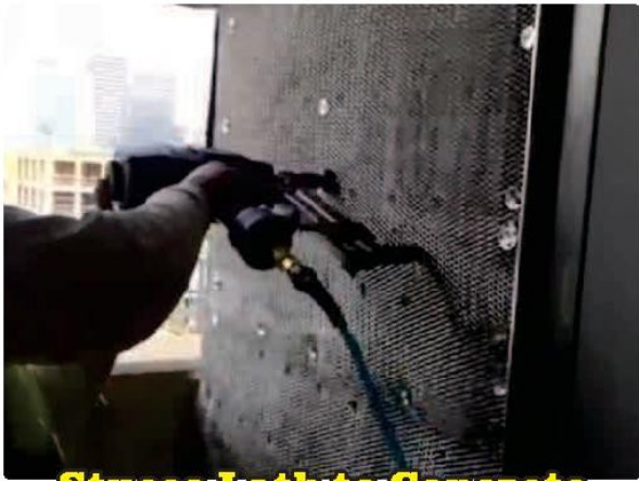
Stucco Lath to Concrete
