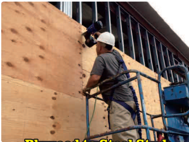
Plywood to Steel Stud
