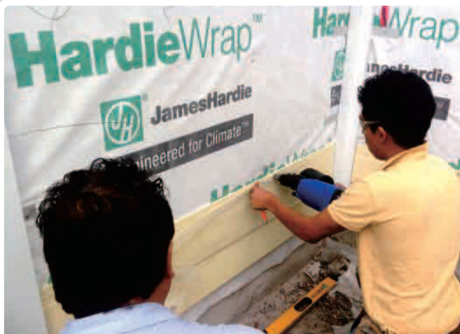
Hardieplank to Concrete Block
